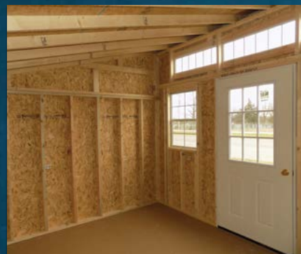
FRAMING SPECS VARY BY LOCAL BUILDING REQUIREMENTS
